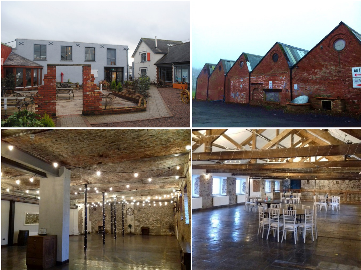
Raceview Mill – from TL clockwise: re-purposed warehouse and residence; post-1890 factory sheds; function room in the wool tower; exposed vaulted ceiling in the wool tower.
