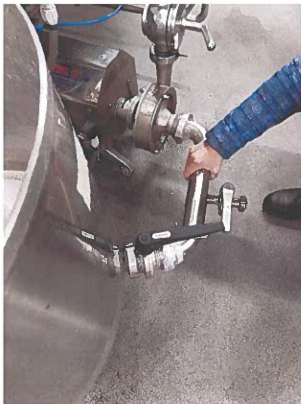
Pipe to be retrofitted so that the waste water can be pumped into an IBC
