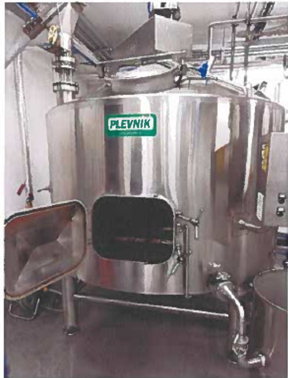
Tank used for first fermentation. Waste product and water were going stright into the drain.
