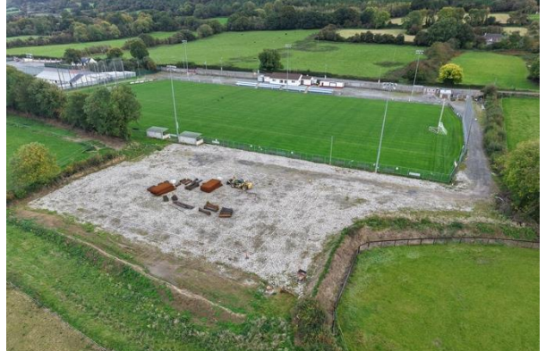
St. Mollerans GAA Ground under development
